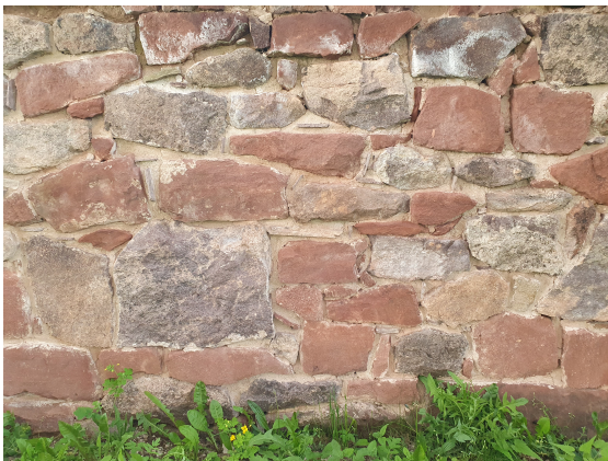
(a) Sample of masonry wall
