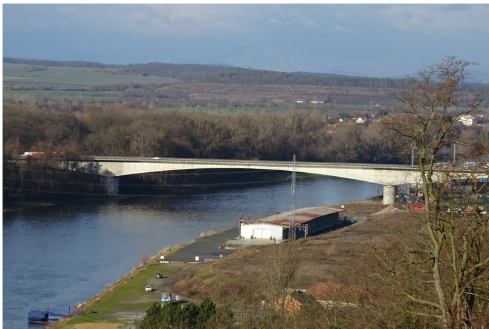
Figure 7.6: Side views on the bridge from the right Labe bank, industrial railway is located on the right side.
