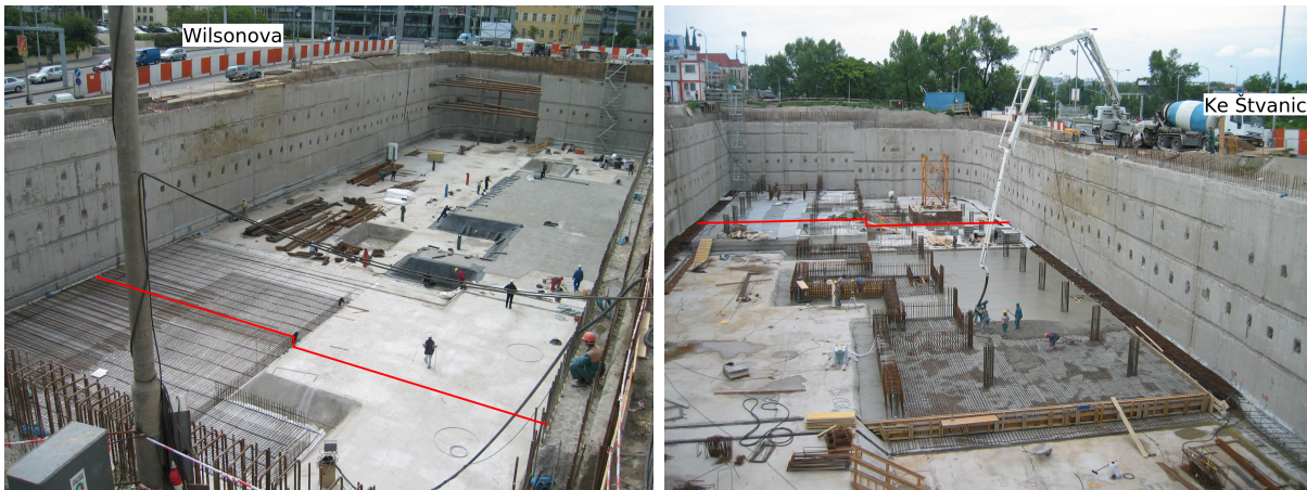
Figure 6.2: View of foundation pit at Těšnov
