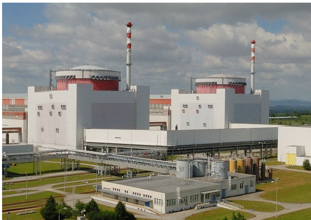
Figure 3.5: Containments in Temelín (source virtualniprohlidky.cez.cz)[CEZ, 2021].
