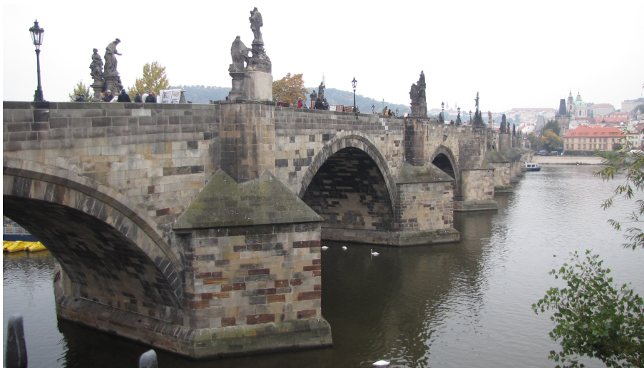
Figure 4.2: Detail of Charles bridge in Prague.
