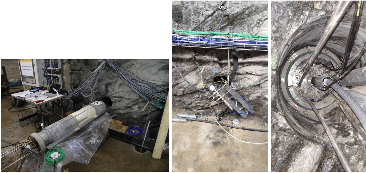
Figure 5.6: Installation and instrumentation of the physical model No. 5 [Svoboda et al., 2019a].
