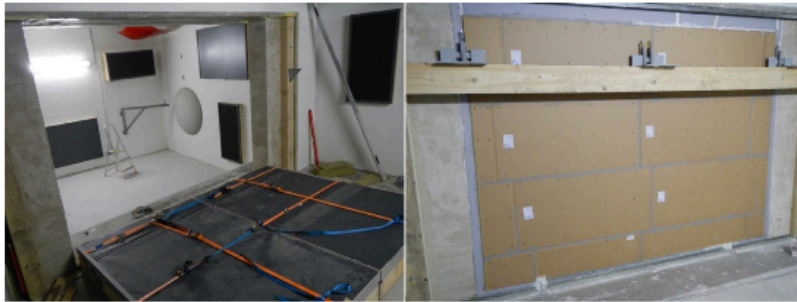
Fig. 8. Installation of the curtain wall system into the test opening in the laboratory (left), test specimen with applied cardboard/sand boards (right).
