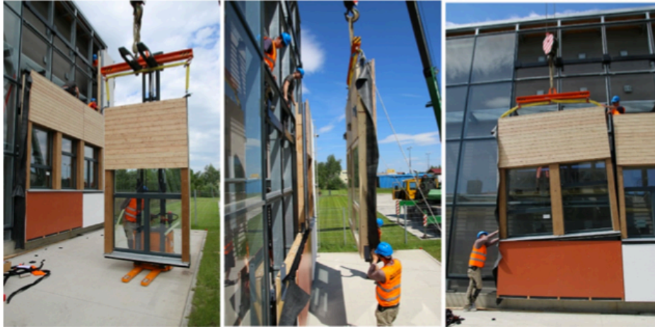
Fig. 4. Installation of curtain wall prototypes.
